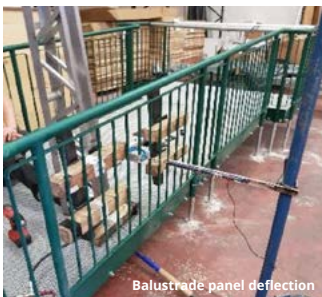
Balustrade panel deflection
